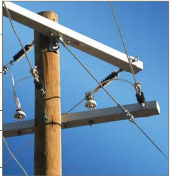
Over 1 million PUPI fiberglass crossarms are at work in a wide range of environments throughout North America and around the world. From hot, wet and dry climates to extreme cold – not a single PUPI crossarm has failed due to environmental degradation.
